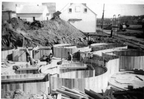
Wood forms for new Co-op storage silos built in 1955
