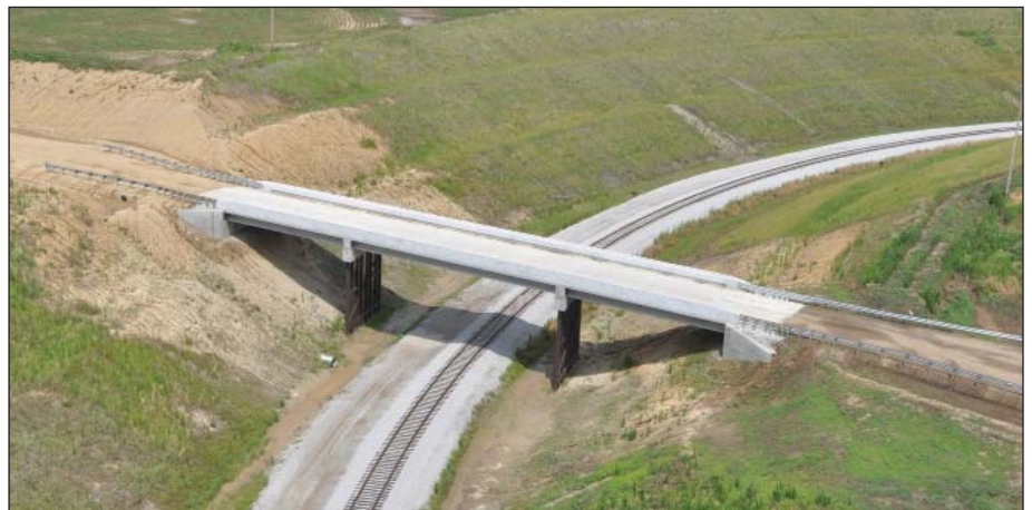
Overpass carries traffic to and from the elevator over a portion of the facility loop track carved into an adjacent hillside. Photo by Ed Zdrojewski.
