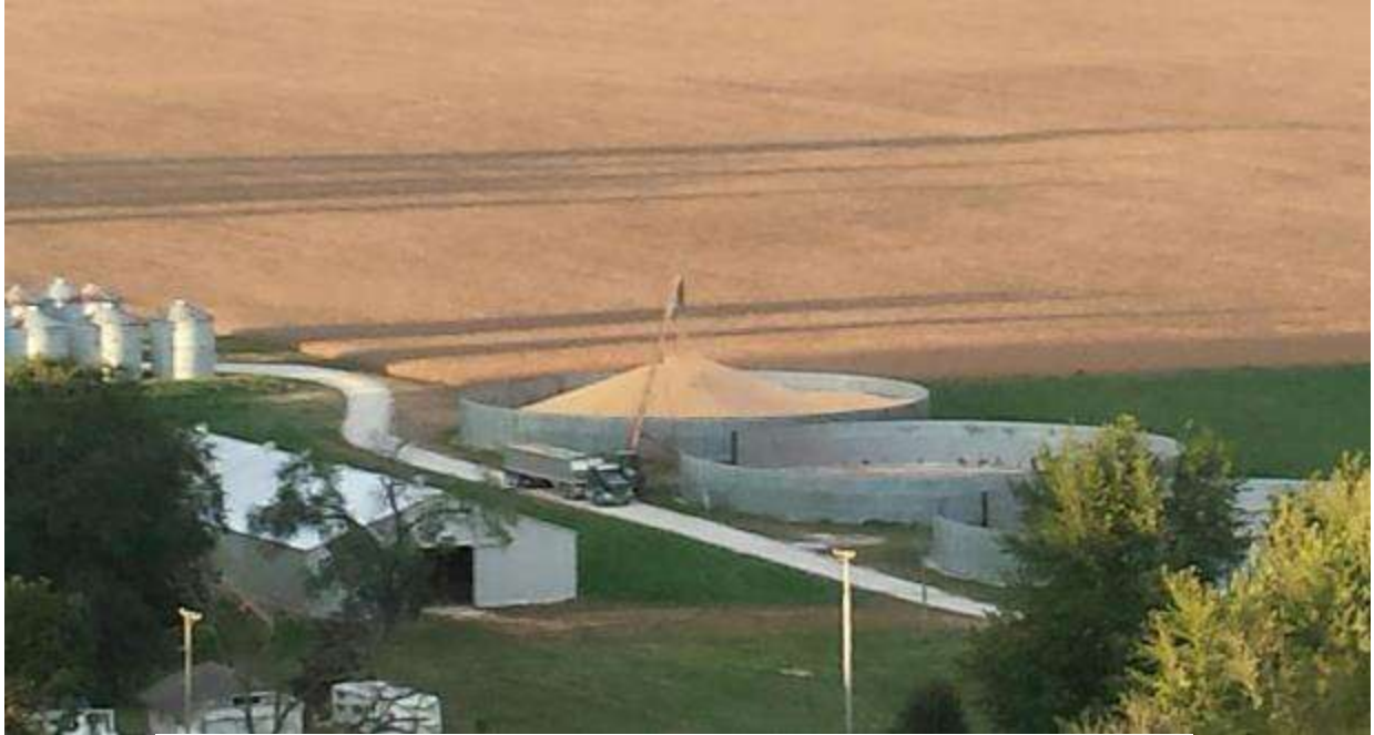
Filling the first Dana Pile
