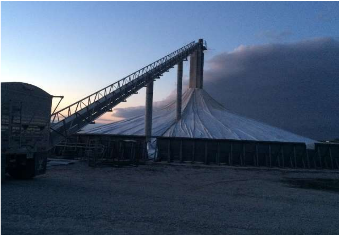
Filling temp pile in Graymont
