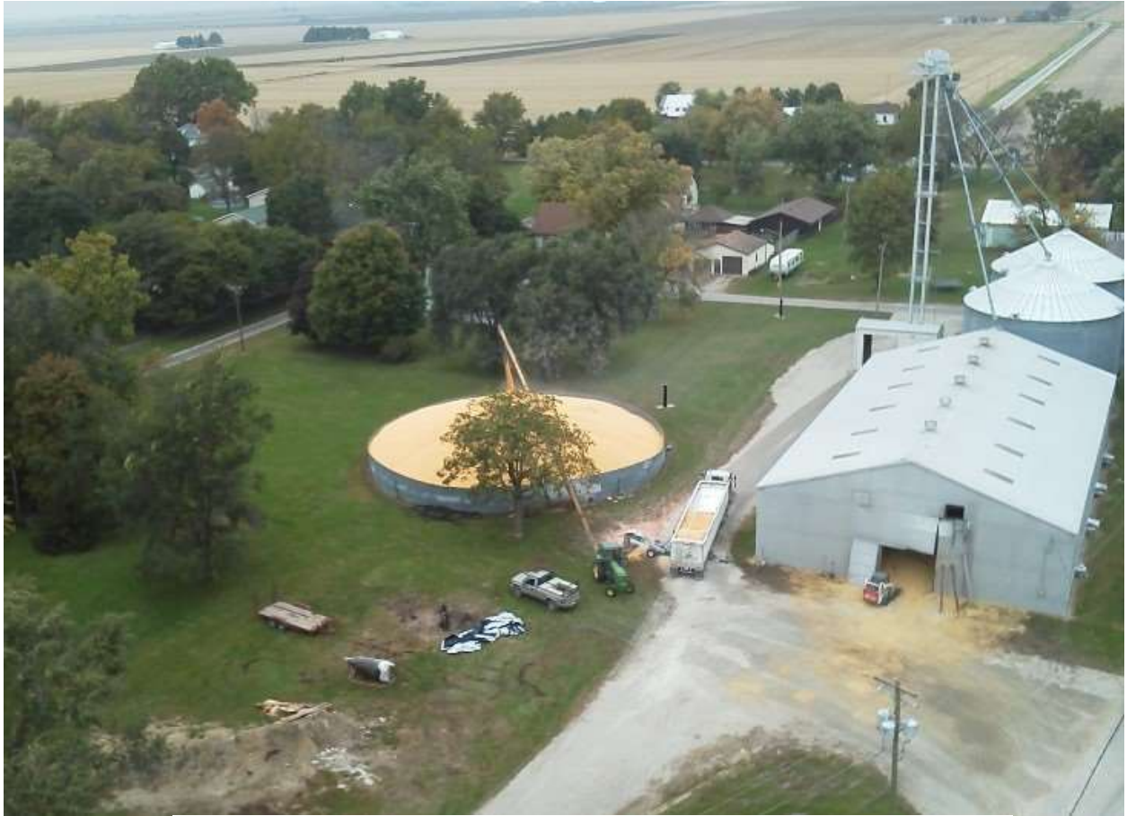
Filling Long Point Pile
