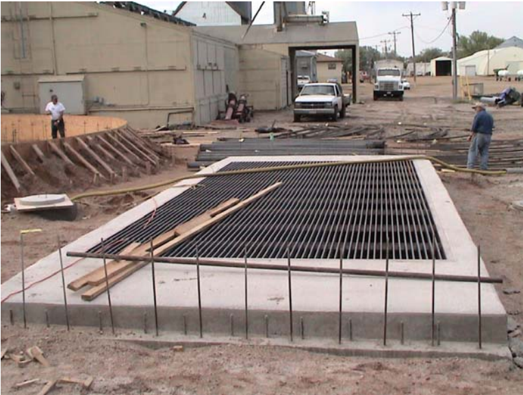
The new dump pit with the grates on.
