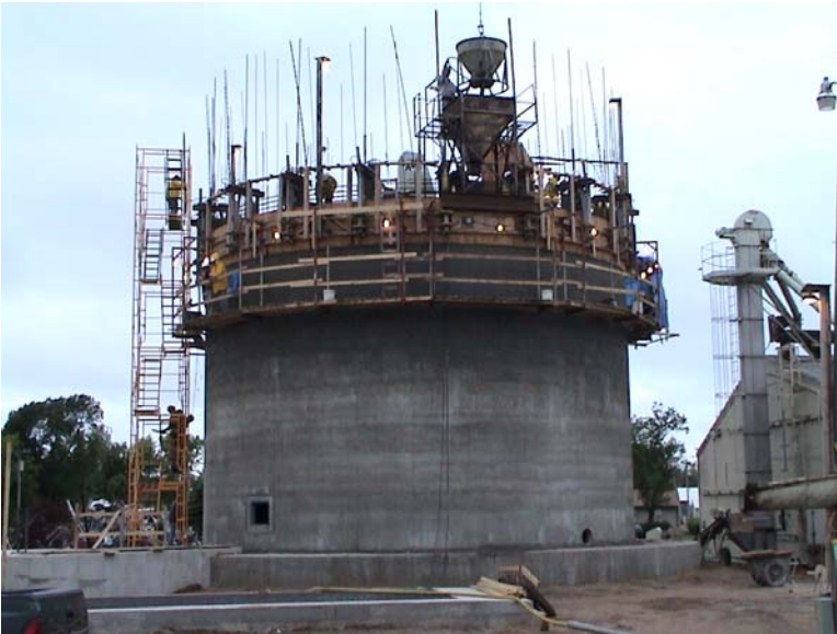
Picture taken Tuesday morning at 7:00 a.m.. The slip was already 29 feet in the air (averaging just over 15.13 inches per hour poured in the first 23 hours).
