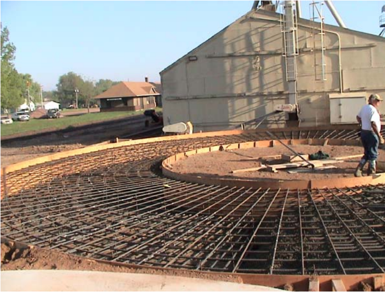
Picture of silo foundation rebar.
