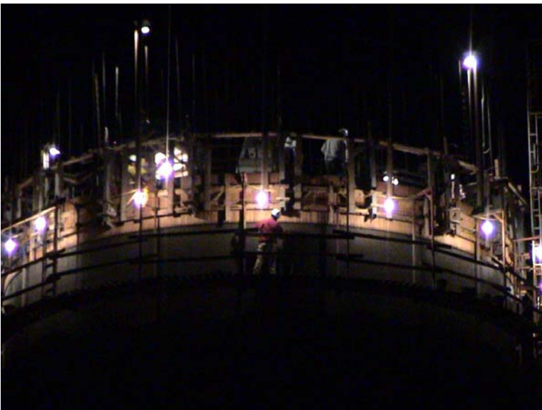
Picture of crew member doing finish work on the slip Wednesday.
