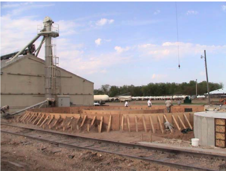
Forming for the donut for the silo foundation.
