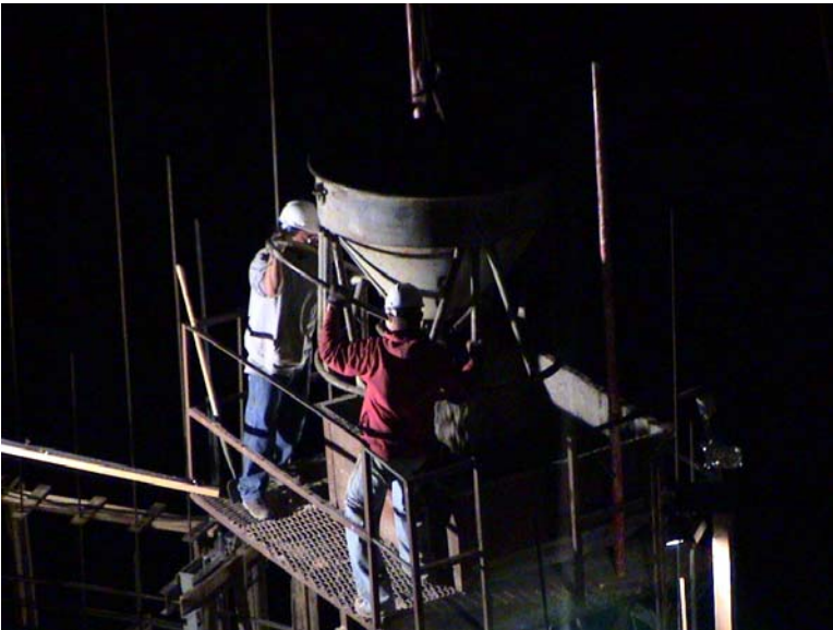
Picture taken Wednesday evening shows the crew working with crane operator to dump concrete in hopper. From the hopper they dump the concrete into carts to move the concrete to the forms.
