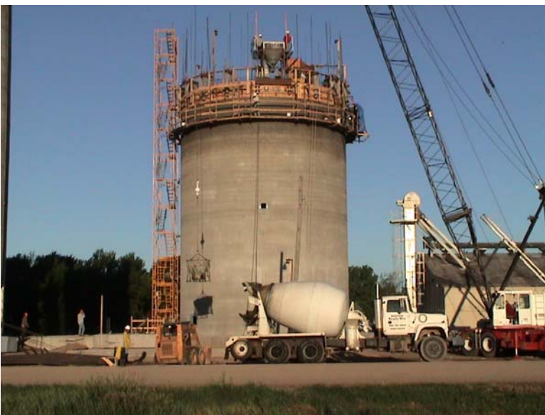
Picture taken 6:45 a.m. Wednesday morning. The slip was 57 1/2 feet in the air. Midwest Elevator predicts that they may be done as early as Saturday morning @ 4:00 a.m..
